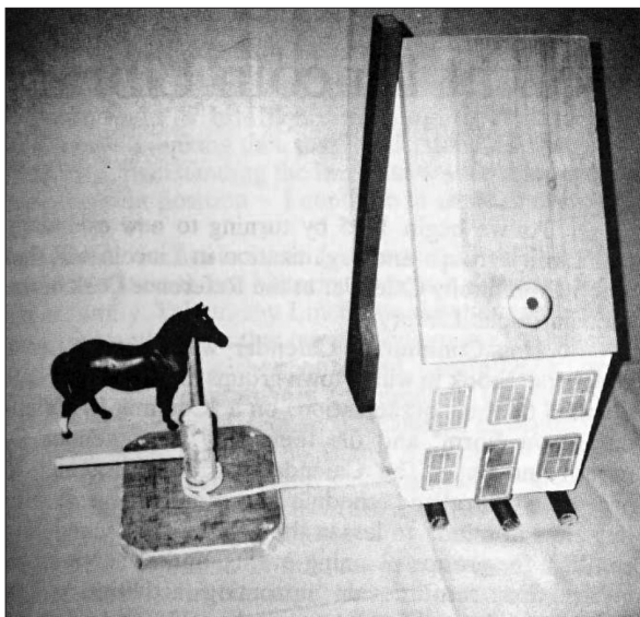
A model made by Warren Flint Sr. shows how houses were moved back in the day. The building was placed on rollers and tied with a rope to a winch, and a horse was pushed a bar to rotate the capstan, thus moving the building 3 feet at a time. (Photo courtesy Lincoln Review)
